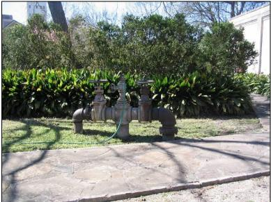
Figure 74. The artesian well at Steve's Homestead has been capped and was accessible for sampling only through a garden hose.
