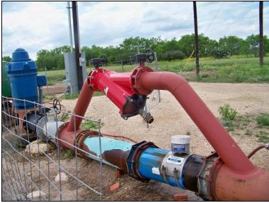
Figure 5. In-line filter sampler.
