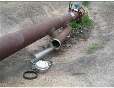
Figure 89. A filter style sampler was installed on the aqueduct outflow at Verstuyft Farms to facilitate easier sampling. The filter is shown here in its disassembled state.
