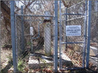
Figure 32. Monitoring Well at Aquarena Center.
