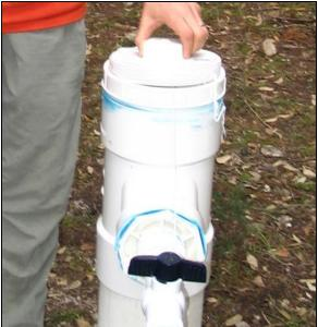
Figure 70. The Schumann Artesian Well is accessed through a PVC pipe.
