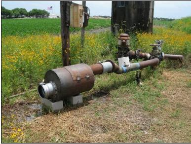
Figure 47. In-line sampler at the Jeff Bailey Well.
